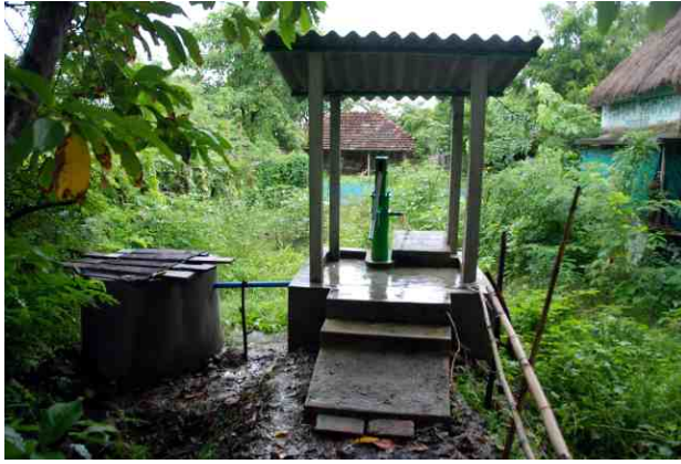
Tube-well Installation for Safe Drinking Water
