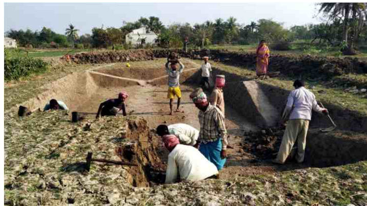
New Pond Excavation for Rain Water Harvesting & Sustainable Aquaculture
